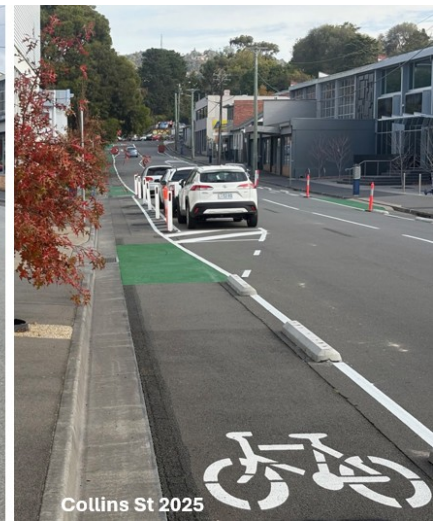
Collins St separated cycleway during installation
