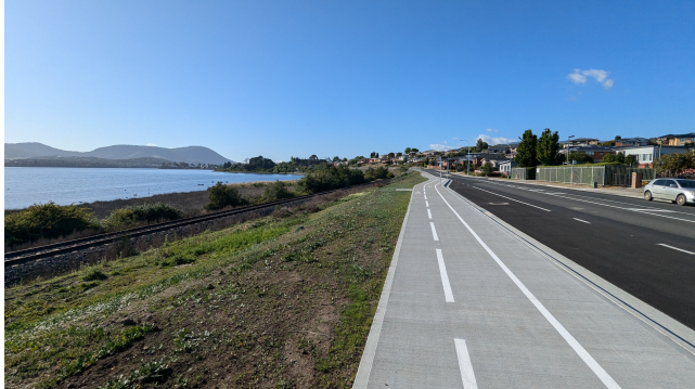
Shared path at Main Road, Granton
