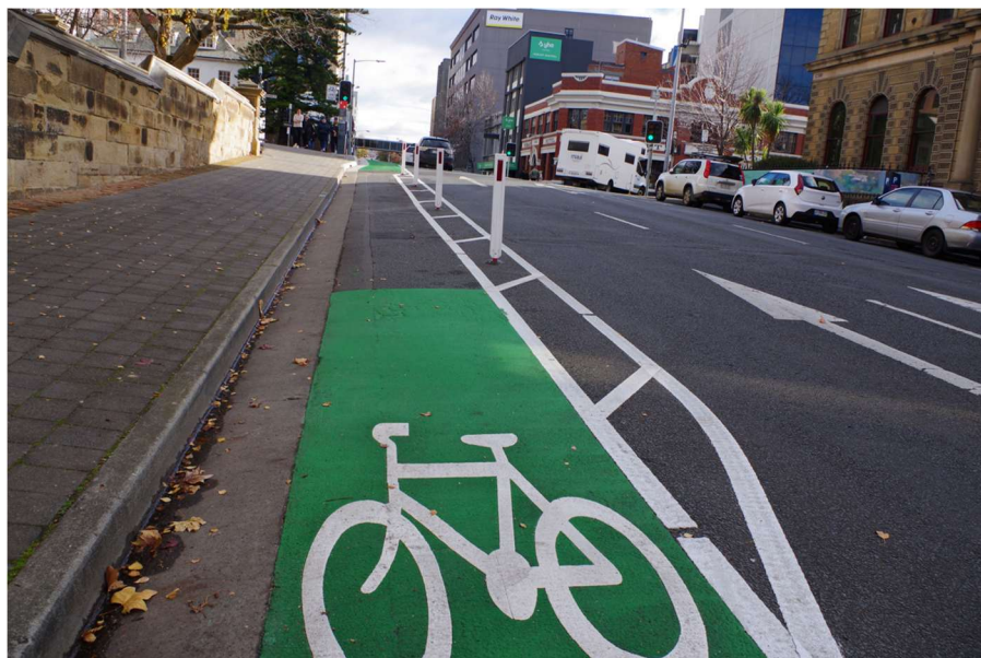
New separated cycleways were installed on Campbell St and Argyle St in 2024.
