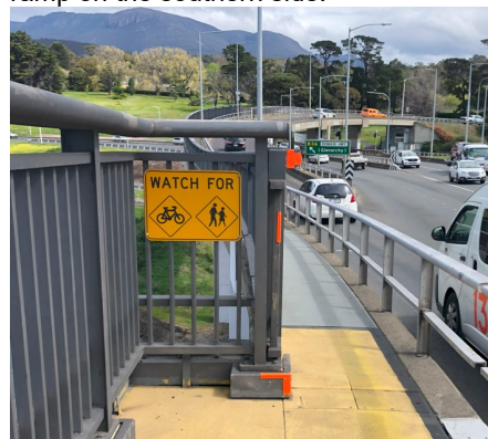
Site 2 - Widen pathway from passing bay to the circular ramp on the southern side.
