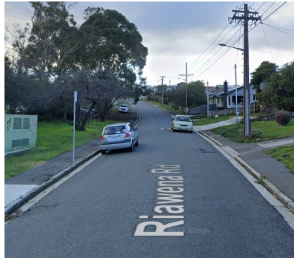
Riawana Road – a narrow road with awkward camber and high degree of on-street car parking. Also a bus route.
